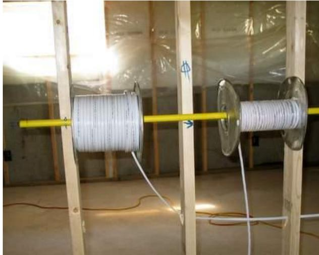
This prevents one spool from unravelling the one next to it. If you are pulling wire in an area that isn't lined up with your improvised wire rack, pull the wire out to a stud space that is, and then pull the wire around toward your workspace.
