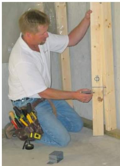
This saves a lot of time, and reduces the margin of error. It's very important to have consistent outlet heights, especially where outlets are fairly close together, like on the backsplash in the kitchen. Tiles will magnify just how bad it will look if the outlets aren't all the same height!
