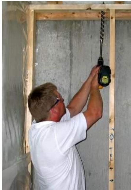
When drilling a series of holes in a long horizontal run, try to pick a nice comfortable height that allows you to use your body to help stabilize the drill and bit. I like to drill the horizontal runs just above hip level.
