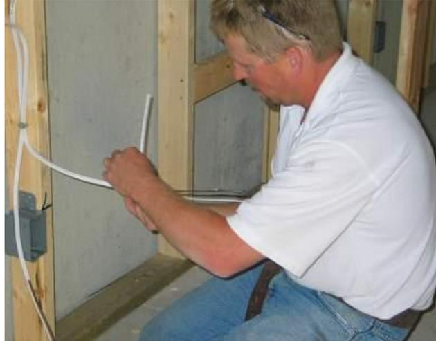
Without some slack, this would necessitate the replacement of the entire run instead of just pulling down the extra cable. It's better to be looking at some extra slack, rather than looking for it!
