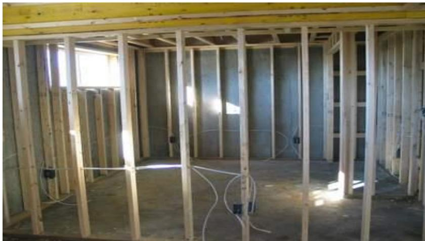
The extra cable above or below the box before tightening the cable clamp is just in case the cable gets damaged somehow before the job is done. All it would take is a careless wall board installer getting a bit too aggressive while cutting out the box openings to damage the conductors or cable jacket.
