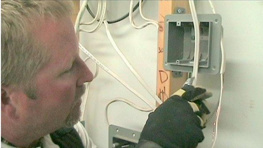
Most arguments to this method revolve around the risk of cutting the insulation on the current carrying conductors, but if you are careful, and gently slide the sharp blade in perpendicular to the wires, you won't harm the insulation.
